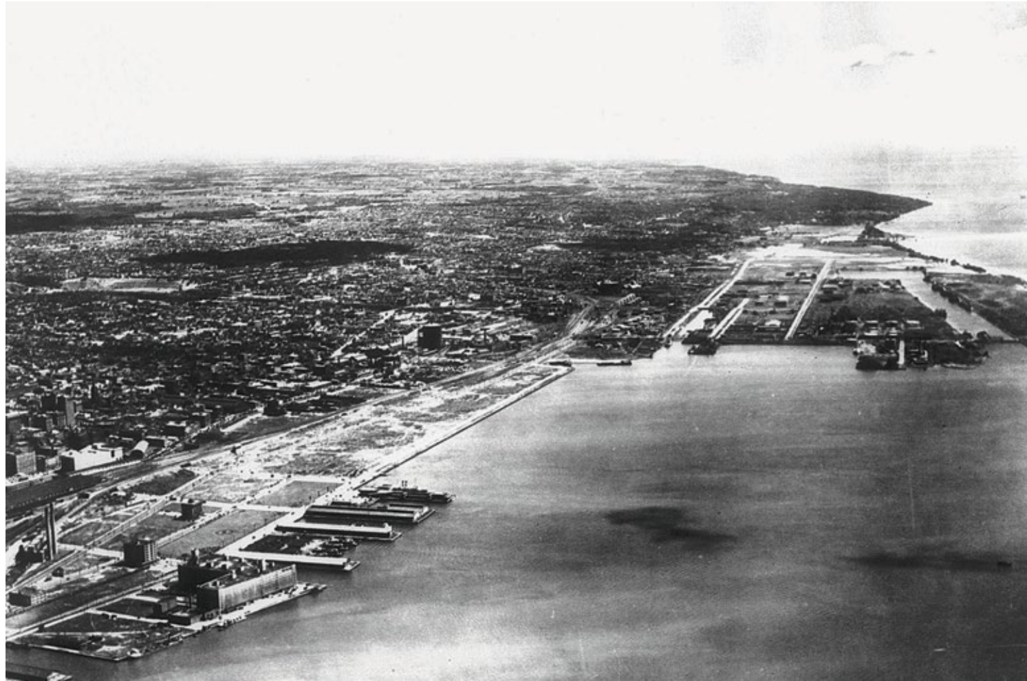
This aerial view of Toronto's waterfront from circa 1933, looking east towards the Port Lands, shows the industrial area created by filling in Ashbridges Bay marsh. Credit: City of Toronto Archives
